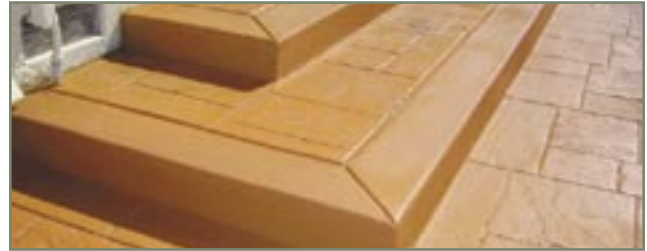
After Freestyle Solid-Color Stain new, fresh looking concrete
