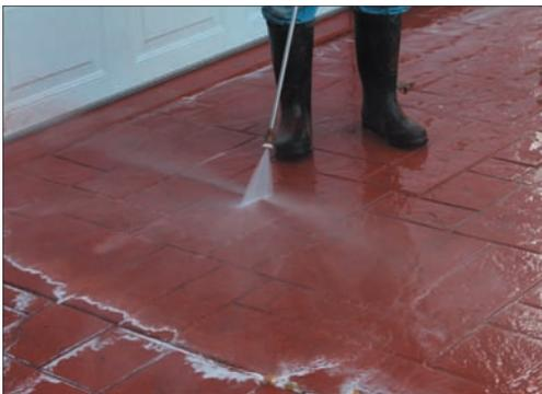
It is vital to make sure the surface is clean and ready to accept pigment. The surface should be free of sealers, dirt, oil, grease, dust, and other contaminants. Furthermore, the concrete should be porous and ready to accept the Antique-It. Use a cleaning and etching agent, such as BRICKFORM E-Etch, to properly prepare the surface.
